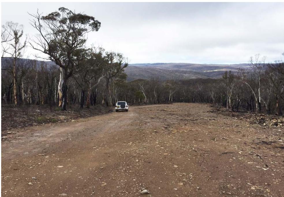
Excessive bulldozer fireline work, which has not been drained or rehabilitated, near Numeralla. (Photo: R. Swain)
